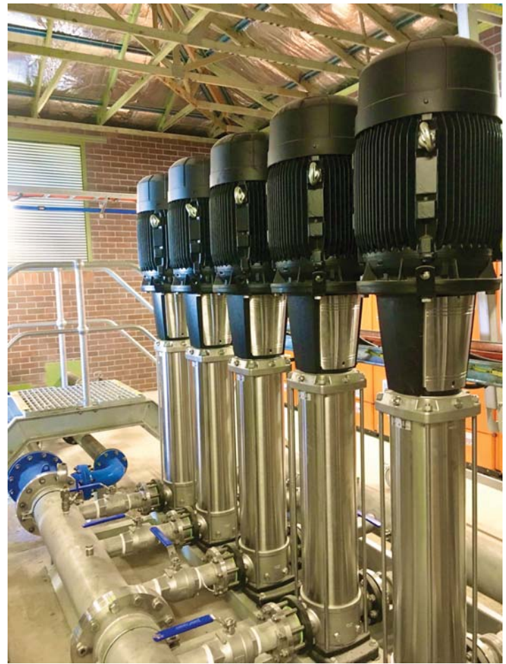
Testing is being conducted on the Malpas Dam pipeline
