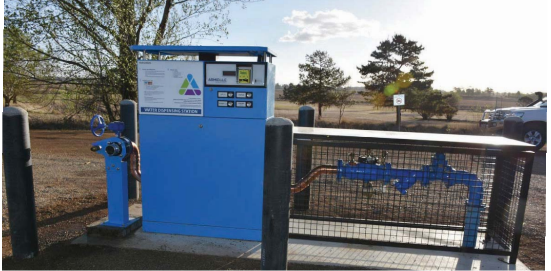
Rural residents can top up their tanks from the water dispensing station
