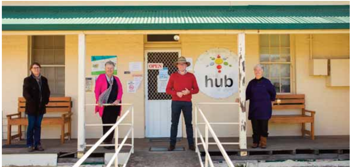
Office Administrator Sonya Shipman, left, Centre Co-ordinator Chris Hietbrink, Adam Marshall MP and President Dot Vickery OAM are looking forward to the expansion works getting underway.
