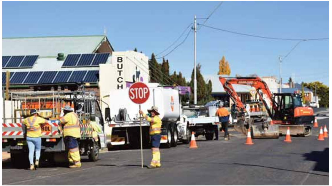
Stage 2 roadworks underway on Tuesday
