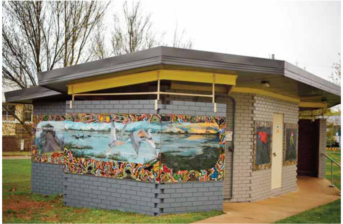
Following last week's unveiling, a fresh coat of paint has been added to the amenities block
