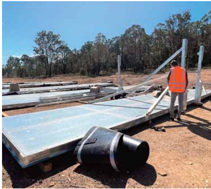
Council staff will be trained in the use of the new landfill lids which will lessen daily soil cover, creating efficiencies and overall saving ten percent of the air space at the Regional Landfill.
