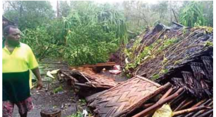
Above: Keskie's home which was damaged during the recent cyclone Left: The house Benoni has built for his family
